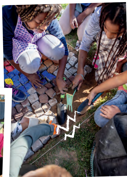
On pose les pavés / Laying cobblestones
