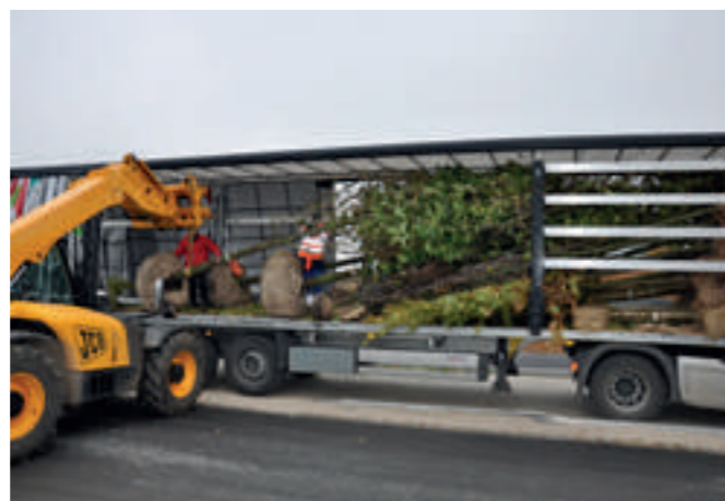
Rue Anatole France in Bonnevoie / Unloading at the building site
