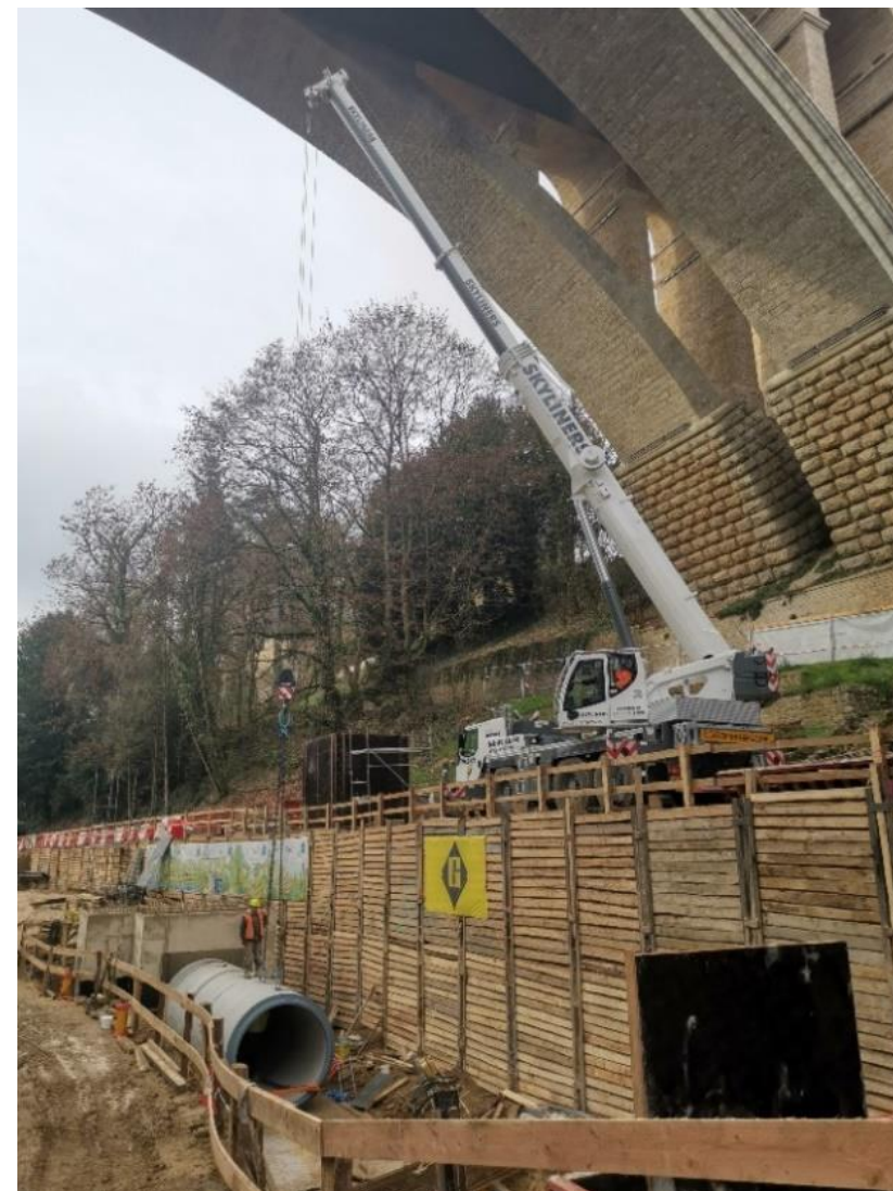
Travaux FIRST FLUSH
